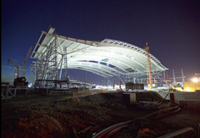
Terminal 5 under construction
